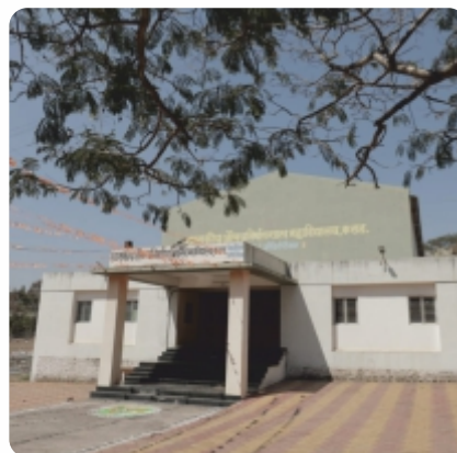
Gymnasium and Sports Complex
